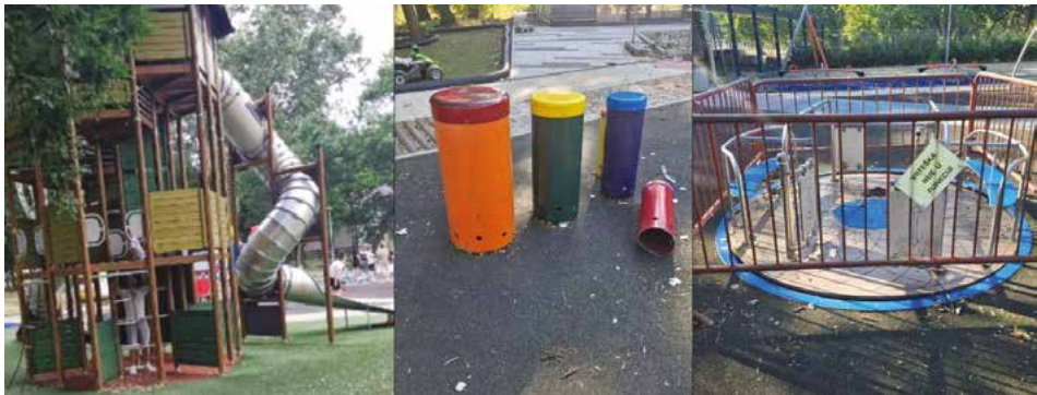
Signs of deterioration and unrecorded additions within the Inclusive Playground during Phase 3
